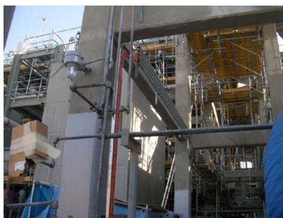
Fig.1 Example of Concrete Fireproofing Application on Structure
