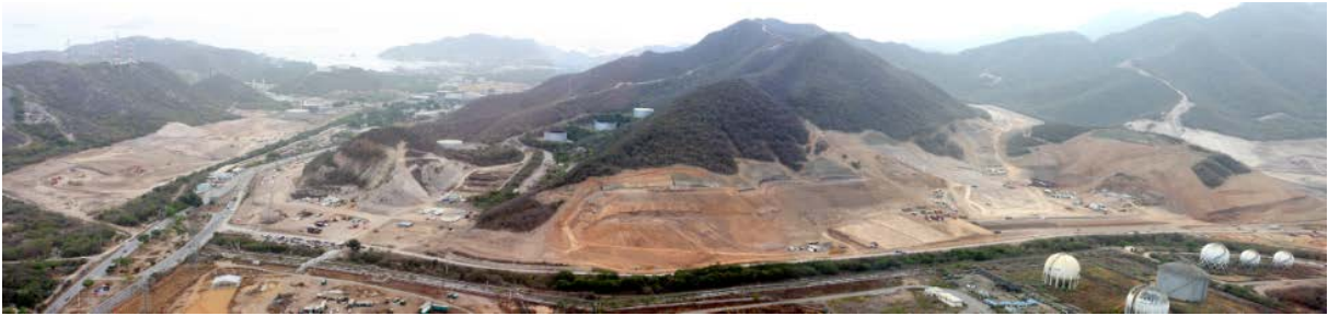
Fig.1 Large-scale site preparation work
