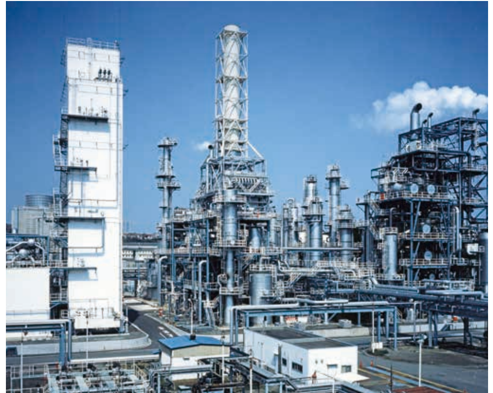
IGCC Plant (Japan)
