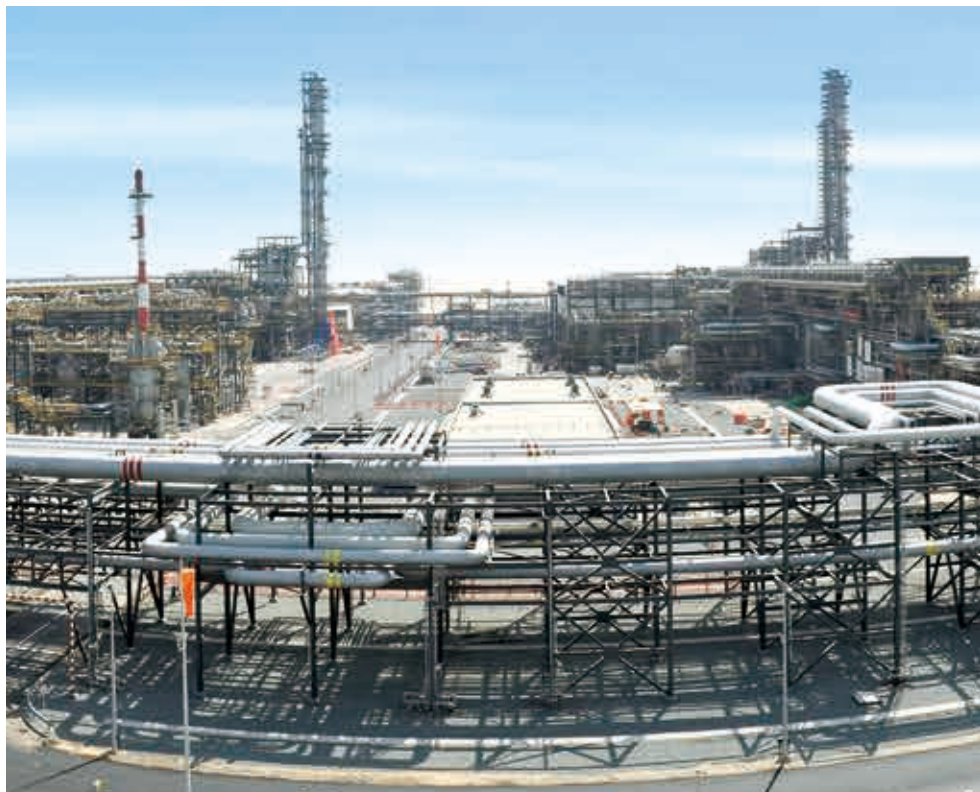
Gas Processing Plant(U.A.E.)
