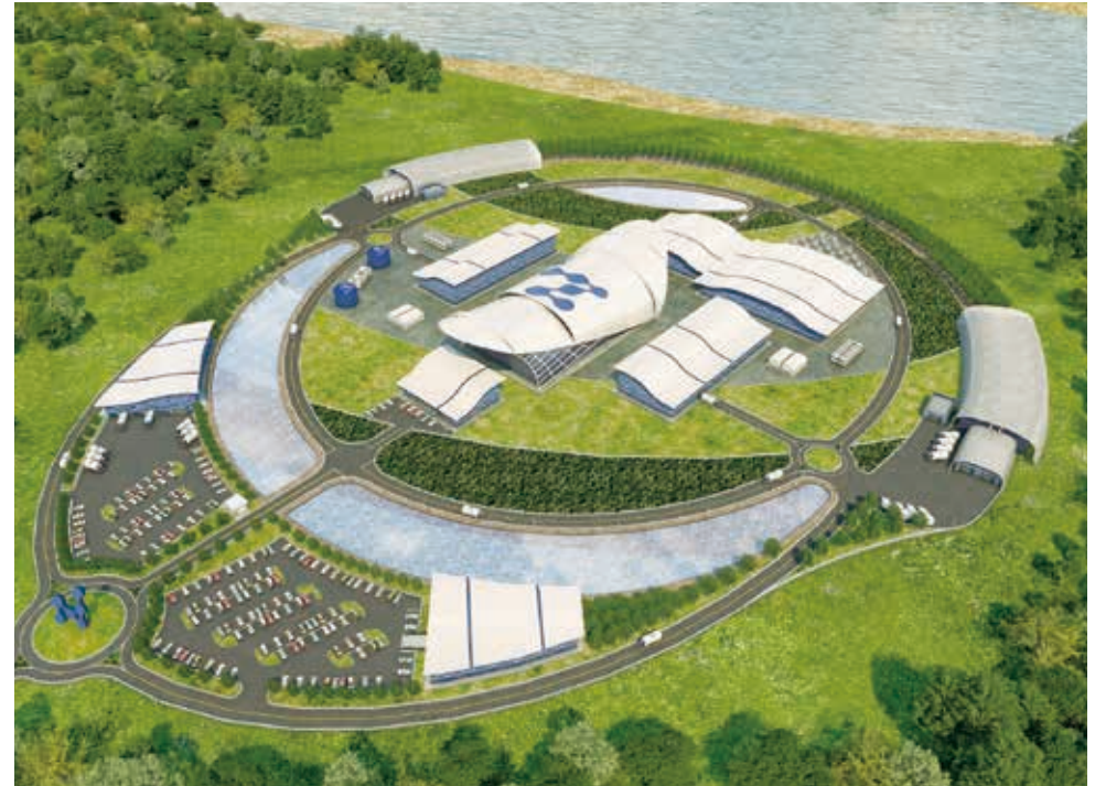
Rendering of the Completed SMR Power Plant Supplied by NuScale Power, LLC
