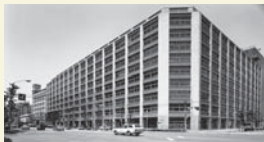
当時の本社 JGC company head office at that time
