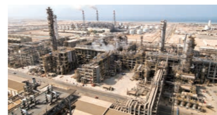
Oil refining and petrochemical complex for Petro Rabigh (a joint venture between Saudi Aramco and Sumitomo Chemical) Completed: 2008
