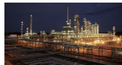
Oil refining plant for PetroVietnam Completed: 2009
