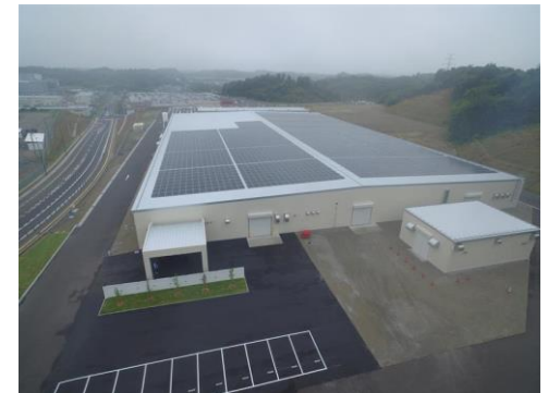
Completed new plant – exterior view
