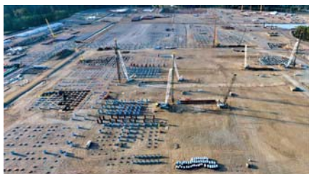
Achievement of major milestone for piling
