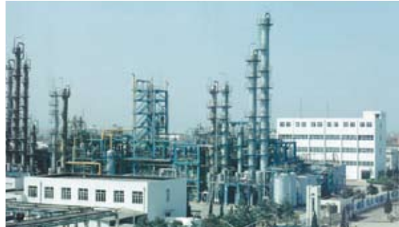
Chlorofluorocarbon substitute production plant (Zhejiang Juhua Co., Ltd.)
