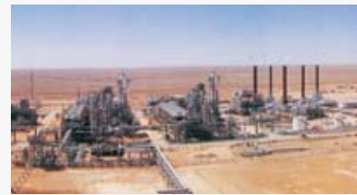
The natural gas processing plant in Algeria
