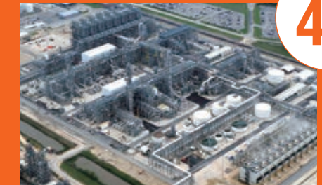
Ethylene plant for Chevron Phillips Chemical
