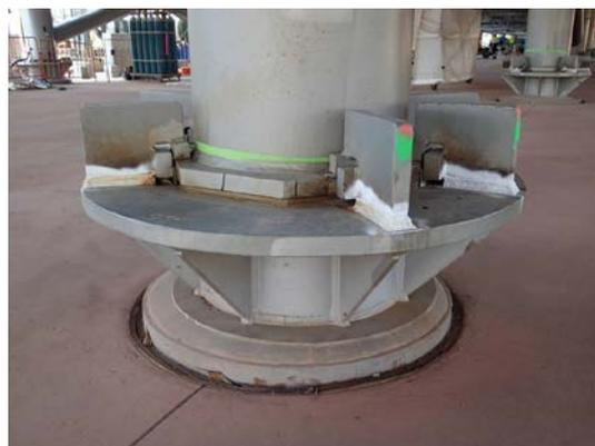
Fig.2 Stab Joint
