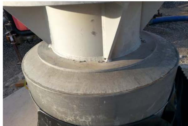
**Fig.6 Finishing Mortar**
