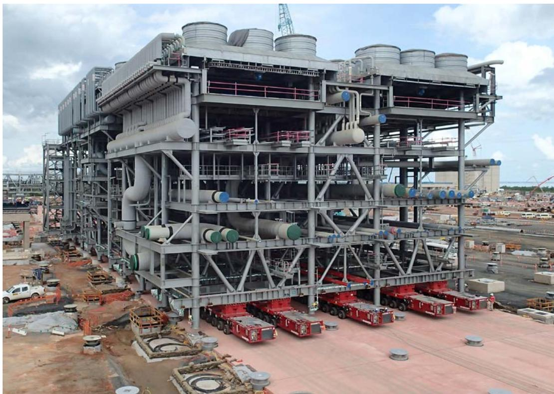
**Fig.9 Big Pipe Rack Module Installation**
