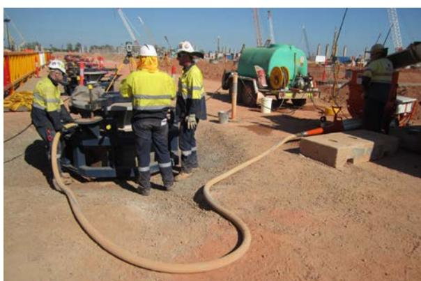
**Fig.5 Pouring of Non-Shrink Grout**
