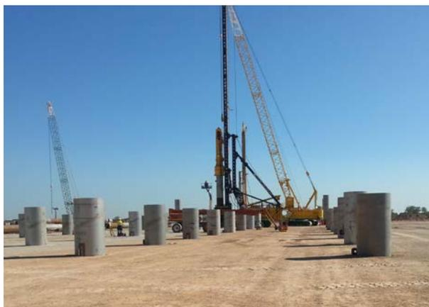
**Fig.3 Pile Driving**
