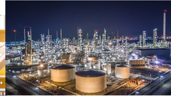
Plant are covered by Fire and Gas Detectors
