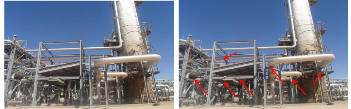
Evaluation of existing Fire Proofing
