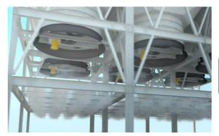
**The water mist** helps lower the air inlet temperature of the ACHE.
