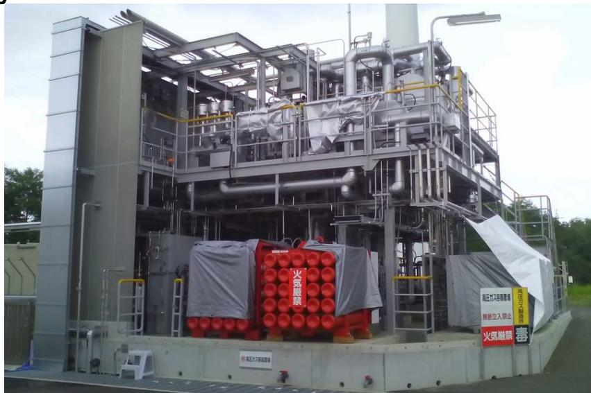
(The red cylinder at the front of the photograph is a high purity hydrogen cylinder storing hydrogen produced from renewable energy.)
