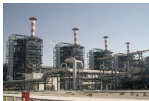
Water and power plant site (UAE, Taweelah area)
