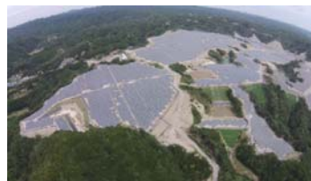
Solar power plant site (Chiba Prefecture)
