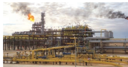
Gas gathering and separation plant for Sonatrach Completed: 2013
