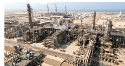
Oil refining and petrochemical complex for Petro Rabigh (a joint venture between Saudi Aramco and Sumitomo Chemical) Completed: 2008
