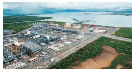
LNG plant for INPEX Completed: 2018
