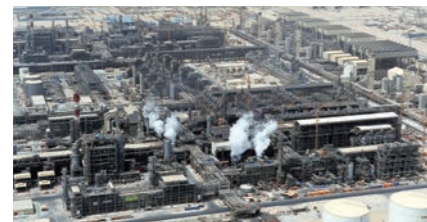
GTL (gas to liquids) plant for Qatar Shell GTL Completed: 2012
