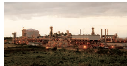
LNG plant for BP Berau Completed: 2009
