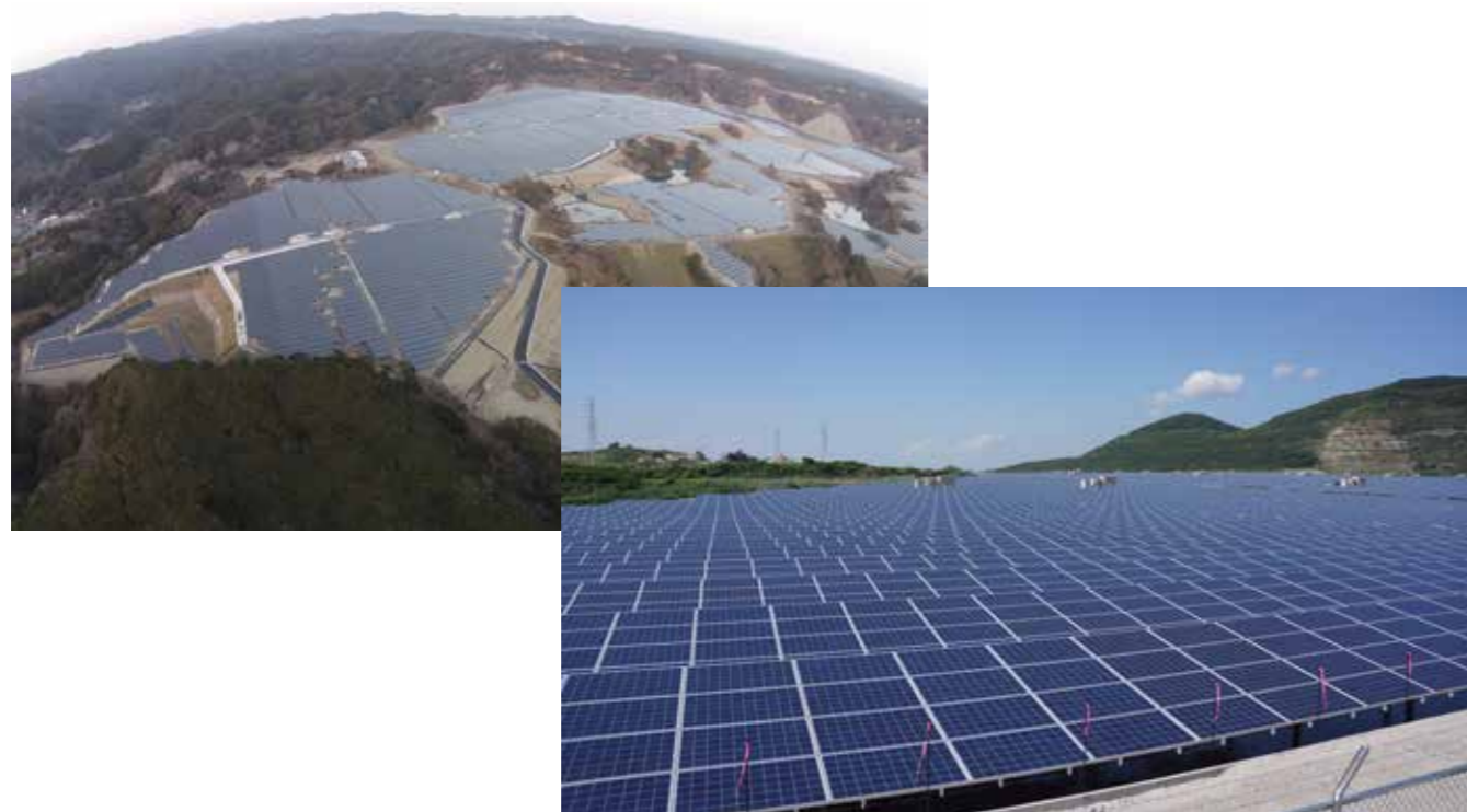
Track Record in Major Renewable Energy Projects
