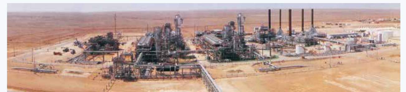
In Salah gas processing plant (2000s)
