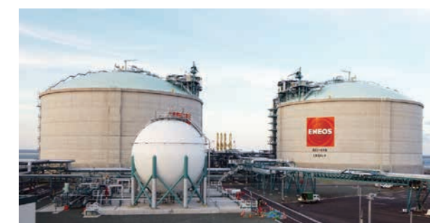
Image: Hachinohe PPG Hiroshi Yamamoto Provided by: JX Nippon LNG Service Company, Limited
