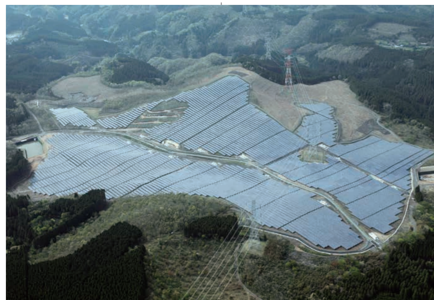
Kokonoe Mega-solar Power Plant (Oita Prefecture)
