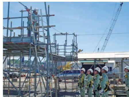
Worksite Training System
