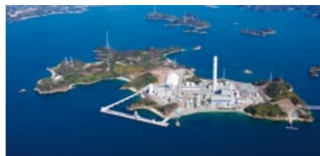
Conceptual drawing of the completed IGCC demonstration plant for Osaki CoolGen Corporation (Hiroshima, Japan)
