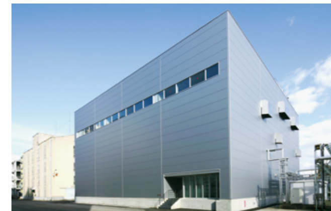
A sterile products plant for TOYAMA CHEMICAL
