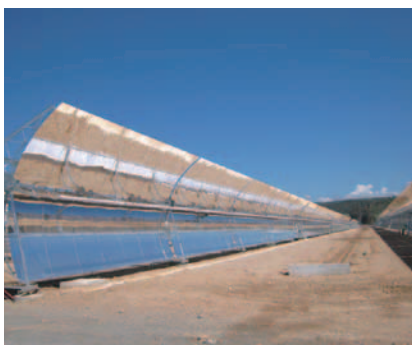
Mirror for concentrating solar heat (photo credit: Abengoa Solar)
