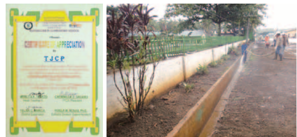
Left: The Certificate of Appreciation from the local community Right: The drainage channel built at no charge
