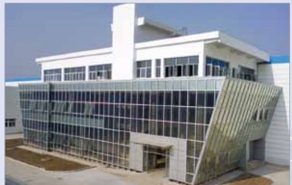
The seawater desalination plant in Tianjin
