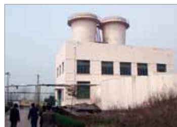
A coal mine VAM duct facility
