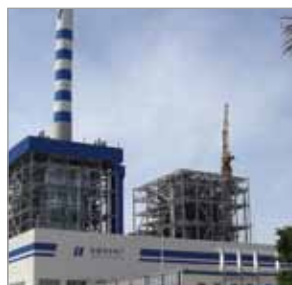
Huaneung Hainan Dongfang Power Plant in China is supplied with NO x removal catalyst.
