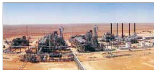
The natural gas processing plant in Algeria
