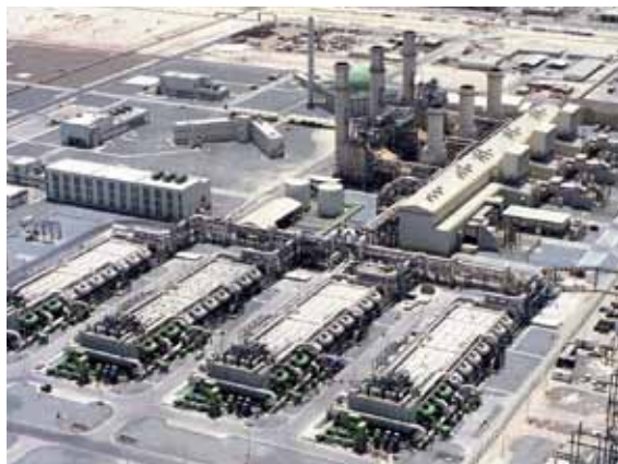
Desalination and power generation plant (Abu Dhabi, UAE)
