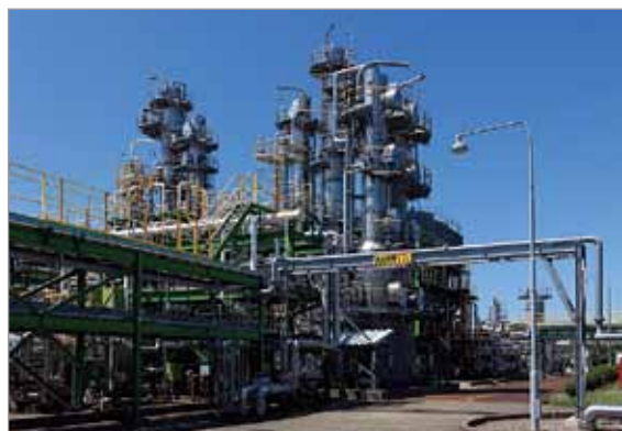
The INPEX Corporation's Koshijihara Gas Plant
