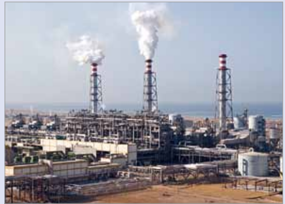
The desalination and power generation plant in Saudi Arabia
