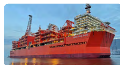
FLNG plant (Africa)
