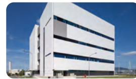
Pharmaceutical plant (Shizuoka)
