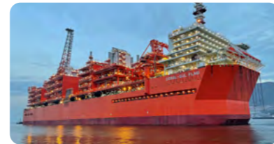
FLNG plant (Africa)
