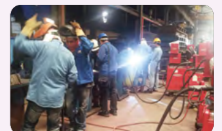
Training for welders
