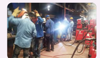
Training for welders
