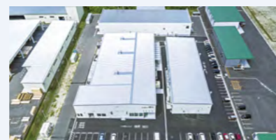
Tomiya Factory, which produces high thermal conductivity silicon nitride substrates and semiconductor production components
